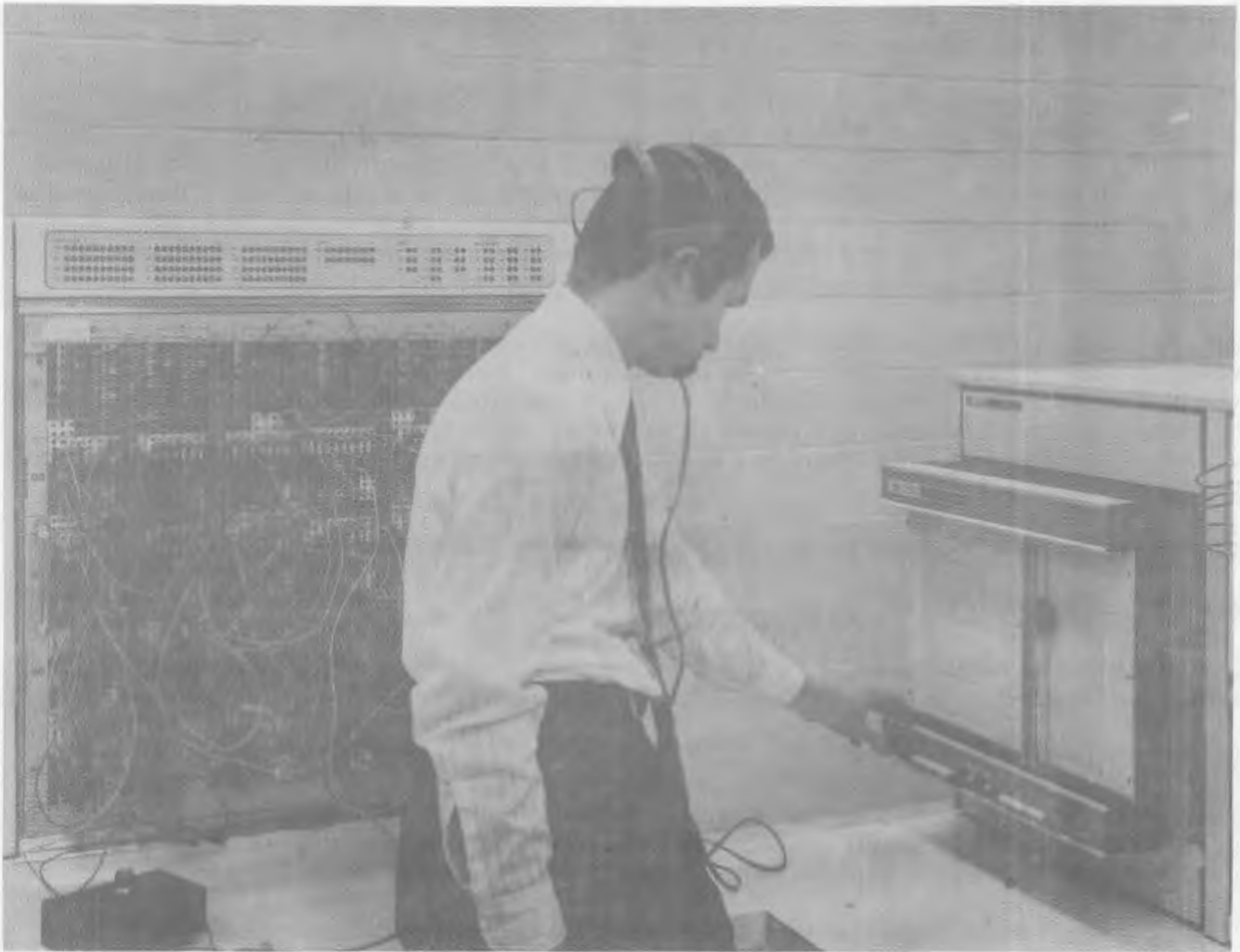
Figure 5-3. Traffic Controller Station.
